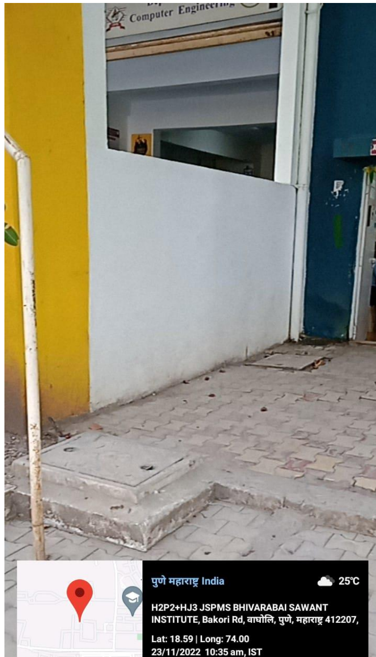
Fig. 6 Rain water storage
